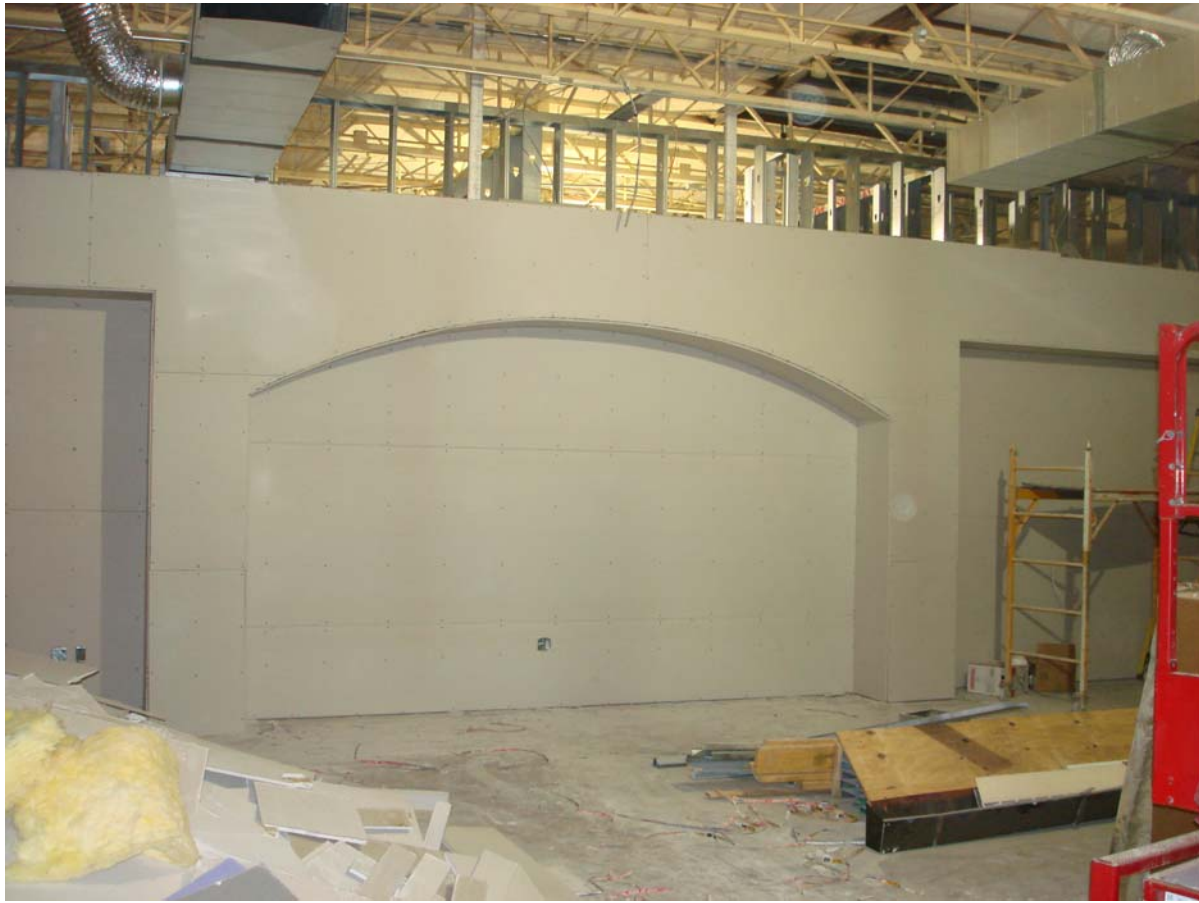
New Classrooms and the small hall are taking shape
